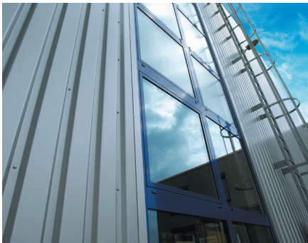
Example of use: facade cladding
